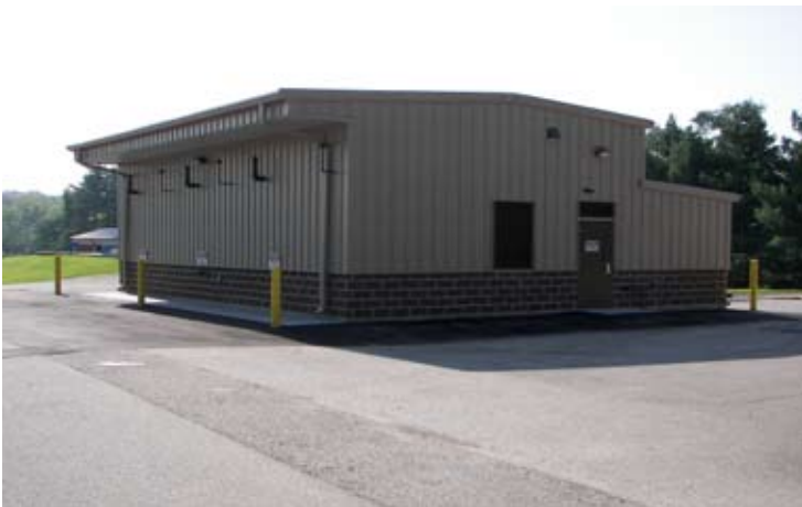
The front of the new Water Works Chemical Feed building
