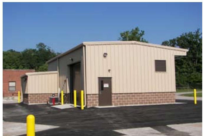
The back of the new Water Works Chemical Feed building
